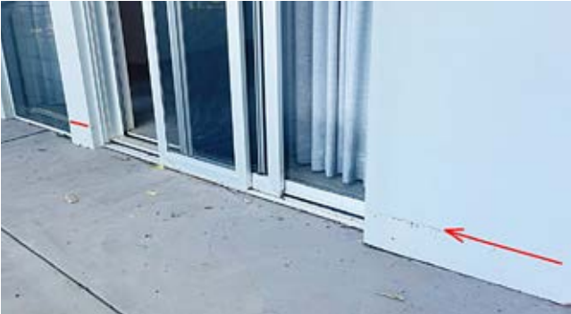
1.574m peak water level at a house in Hay Ave (red lines added for clarity)
